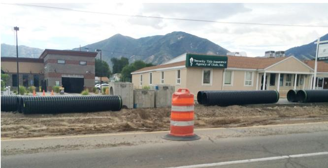
Additionally, the pipe's structural capacity to withstand vehicle weight has been proven under Cooper E80 Loading conditions.
